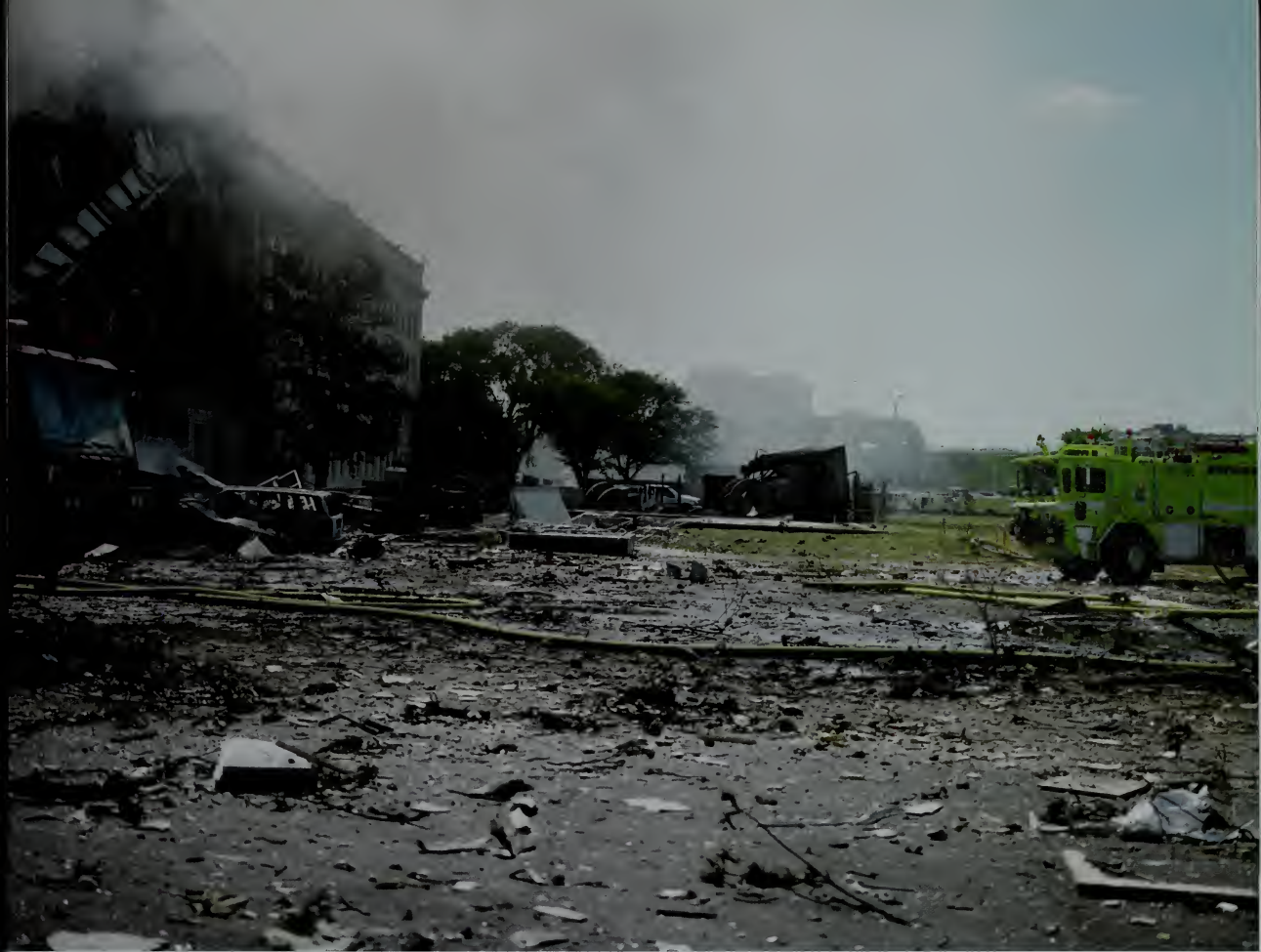
Above: Debris covering the Heliport area.
